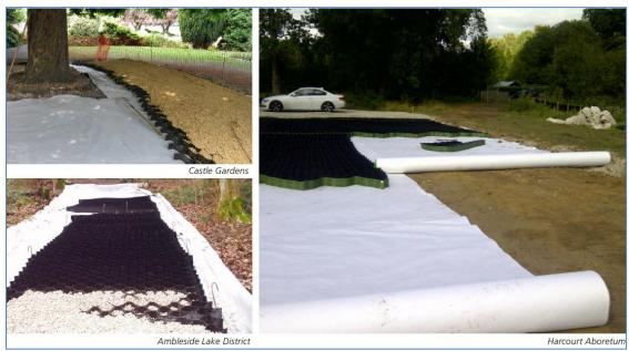
Figure 3: example cellular confinement system.
